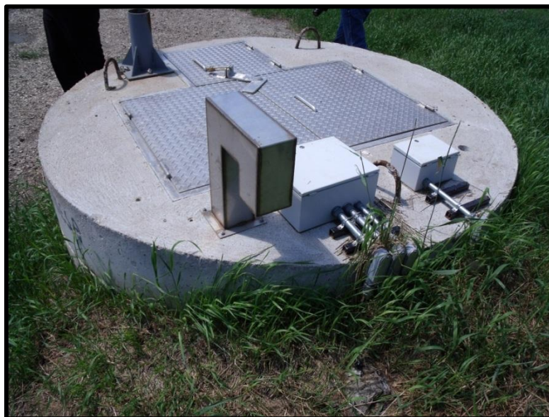
Figure 2: Wawanesa Lift Station Exterior
